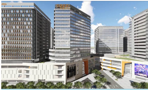
Nangang Rail Yard Shopping Mall (In Progress)
