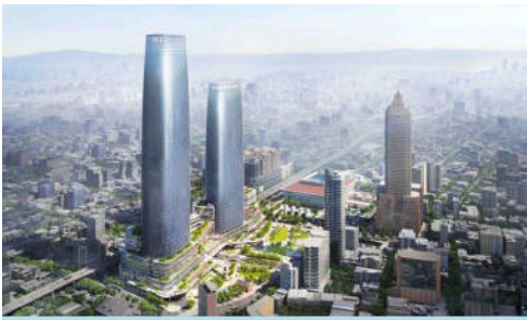
Taipei West District Flagship Project (In Progress)
