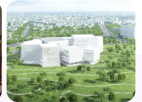
Taichung Public Library, Taichung Art Museum (In Progress)
