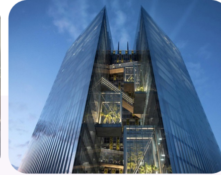
Taichung's 7th Redevelopment Zone Ultra Five-Starred Brand Hotel (In Progress)
