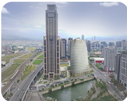
LIHPAO Group's Xinzhuang Headquarters Building
